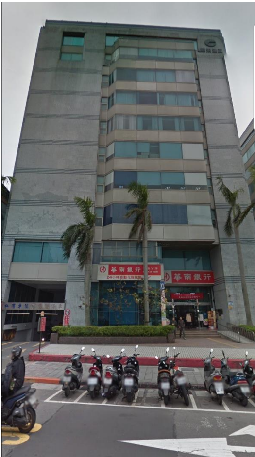
Figure I. 3. Building Office A
